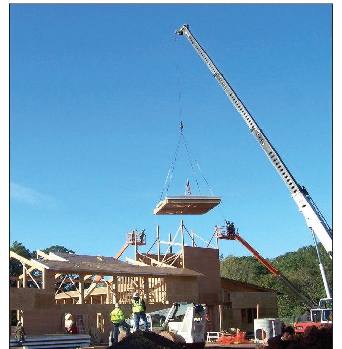
The Kohler Center at Choate under construction
