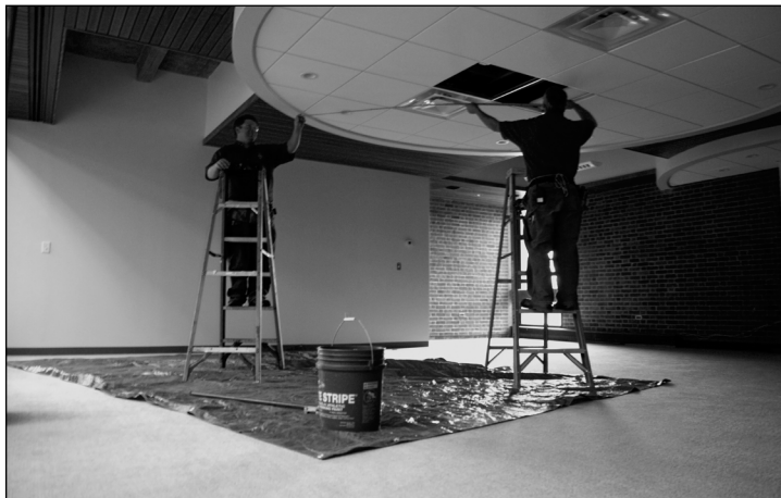
The new Kravis Center under construction
